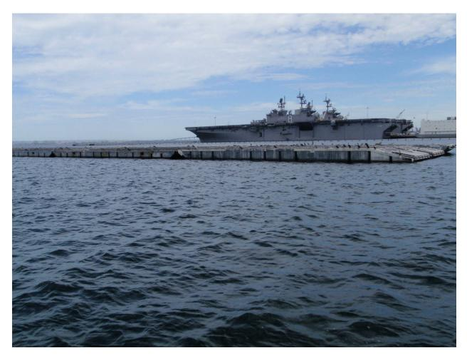
The 45' x 7' barge sections are transported to the site on tractor-trailers, then assembled in the water.
